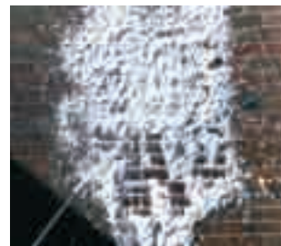
Apply high density foam to large areas quickly.
