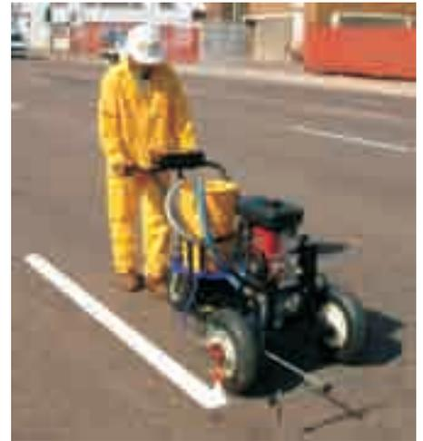
The Hawk 4200 road marker can also be used for conventional spray painting, by simply detaching the gun from the line-marker holder. It can then be used for stencil work or any other coating application.
