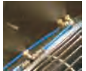
Nozzles mounted on fan for fogging purposes.
